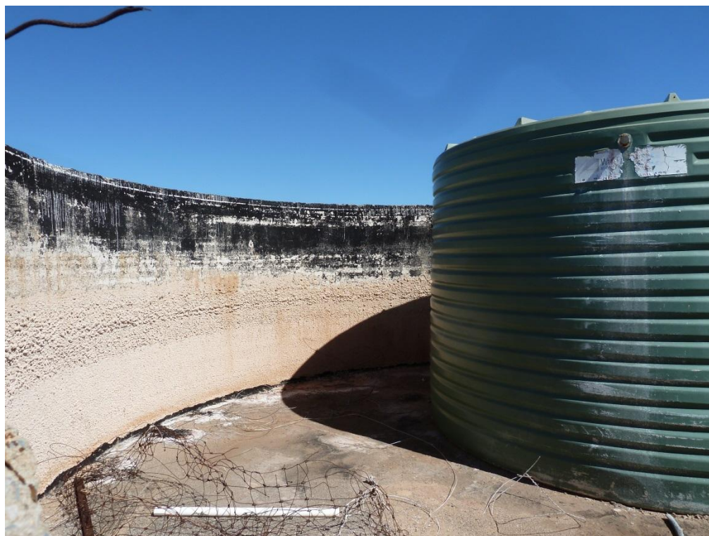
Plate 2 Newer water tank inside of concrete exterior
