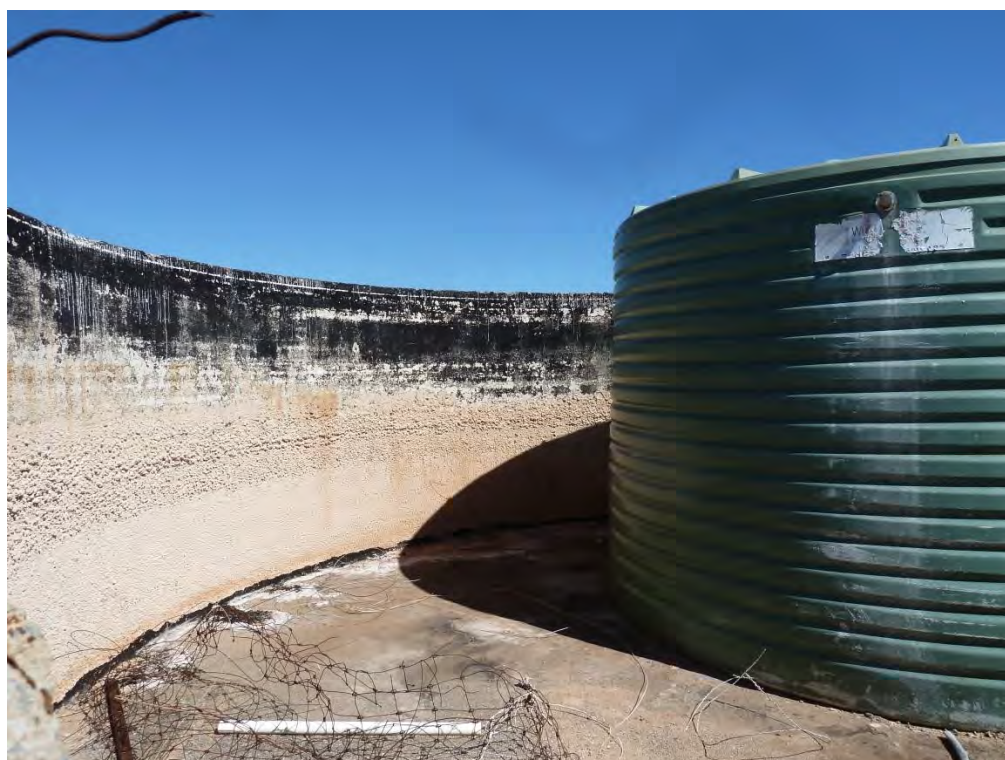
Plate 2 Newer water tank inside of concrete exterior
